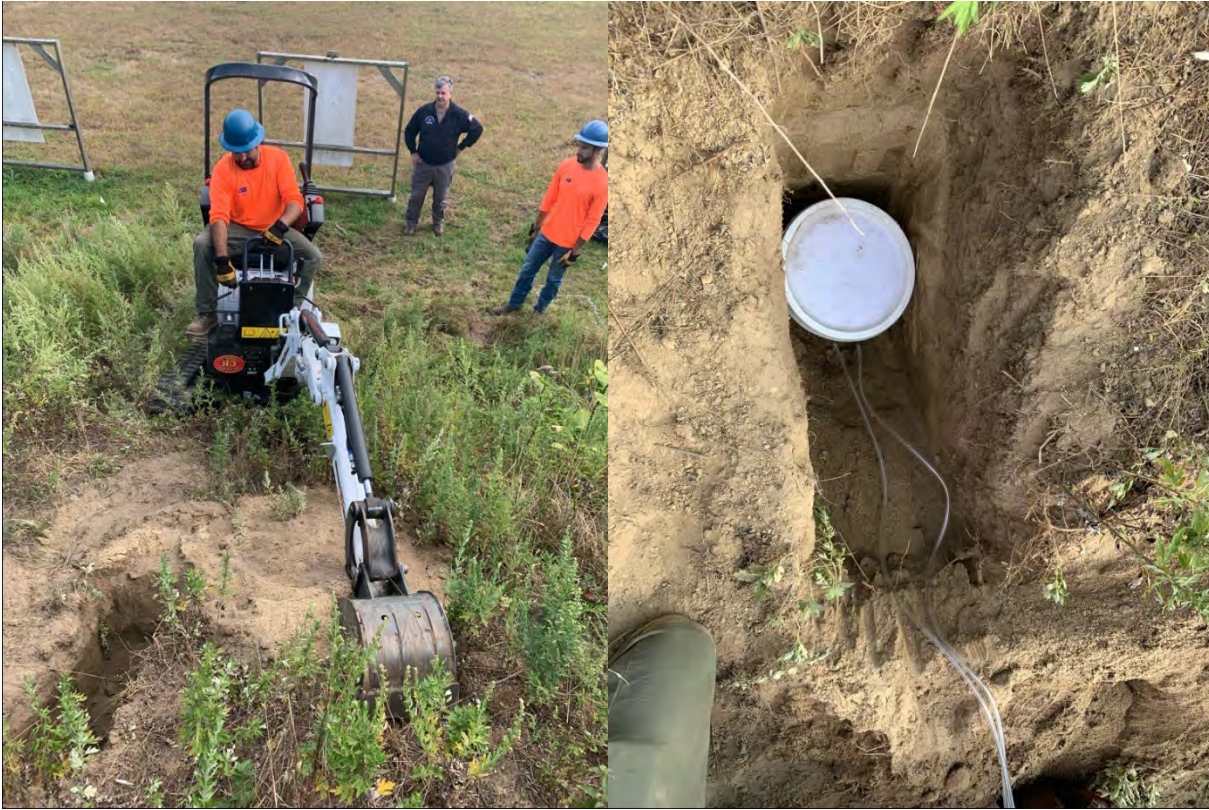
Lysimeter installation under a bullet pocket on the India Range backstop berm. Photos by MANG Environmental & Readiness Center
